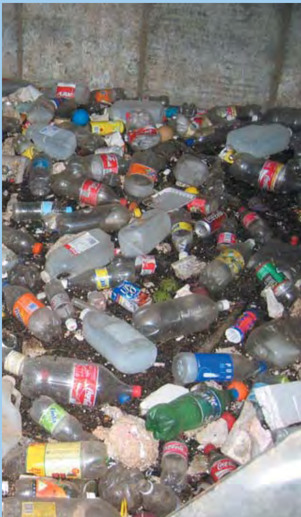
Rubbish and debris captured and retained inside a Humegard™ unit
