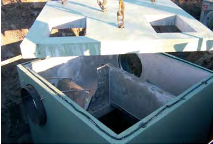
Placing the lid on a Humegard™ installation
